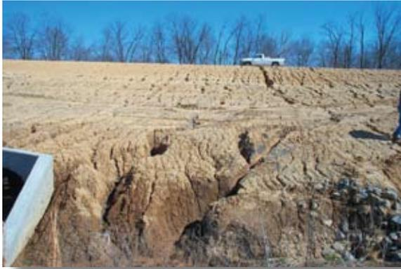
*Long, bare slopes need to be stabilized. Polyacrylamide offers excellent temporary protection for slopes that will not be seeded or mulched immediately. Do not use near creeks, rivers, or wetlands. Follow manufacturer's instructions.*
