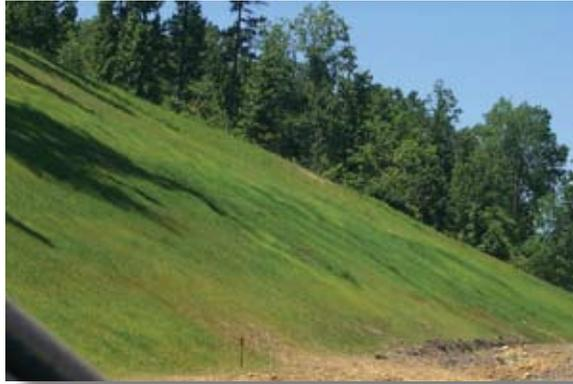
*Establishing grass through broadcast or hydro-seeding reduces erosion and sediment loss by more than 90 percent. Use mulch on short flatter slopes and erosion control blankets or hydro-mulch on long steep slopes.*
