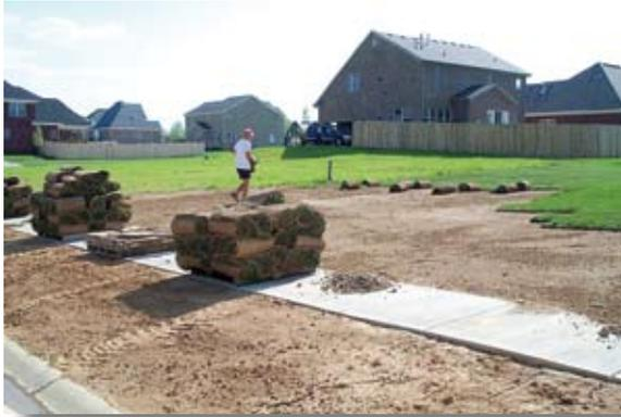
*Sod reduces erosion potential to near zero. Make sure the surface is properly prepared with appropriate soil amendments; use fresh sod and keep well watered during the first 2 weeks after application.*
